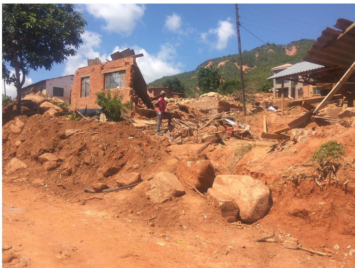
Houses damaged in New Stands Village in Chaimanimai District
