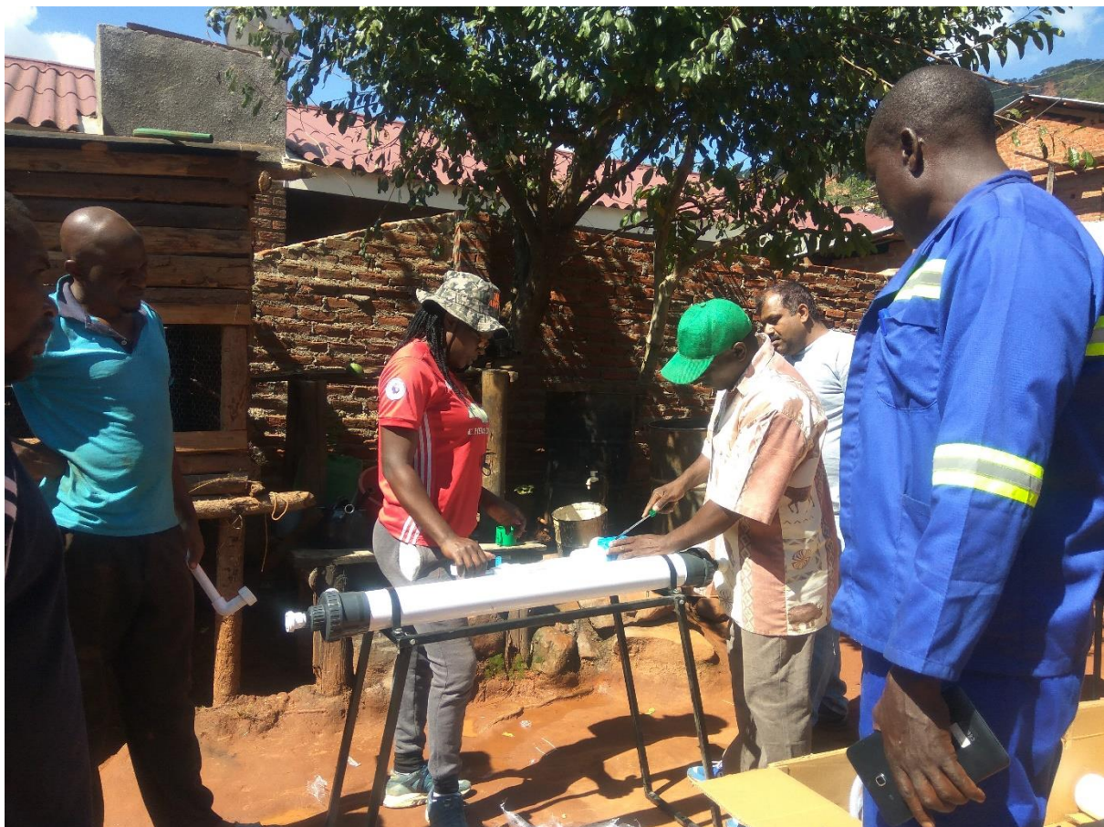
Water filtration plant installation by ZUNA team
